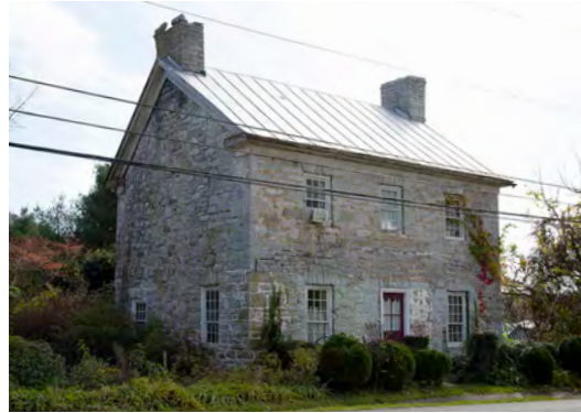
Keezle House, photo by Chris Anderson
