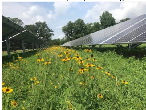
Gold Certified Cople Elementary School Solar Facility in Westmoreland, County (developed by SunTribe). Photo is after first growing season.
