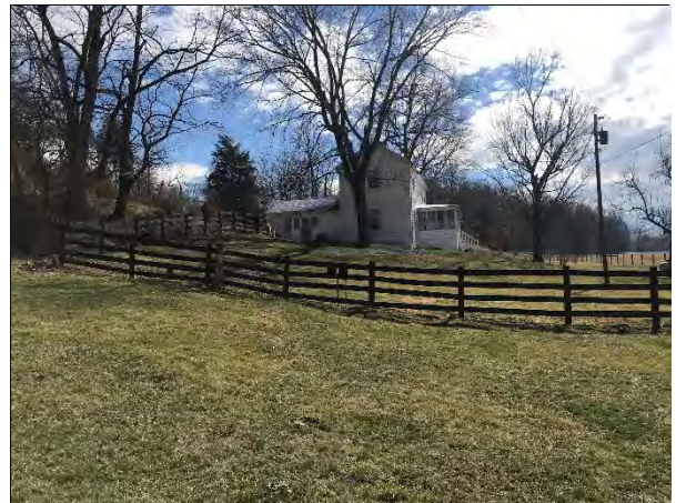
House in the southern area of the Site
