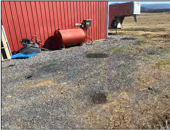
AST and light petroleum staining near the farm buildings near the western boundary
