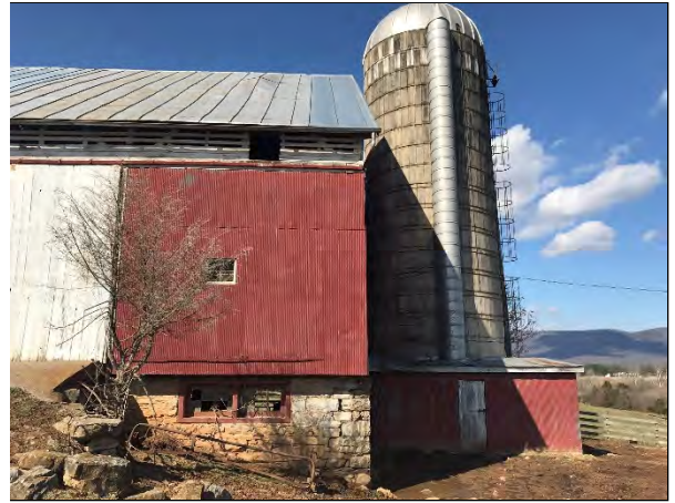
Farm structures at the northernmost farm on the Site
