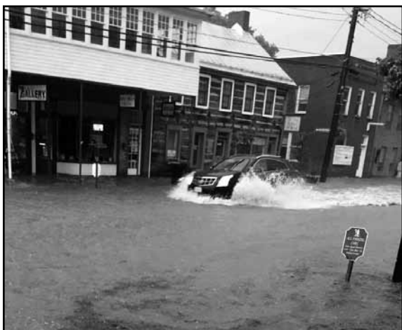
On July 13, 2015, a torrential rain storm, bringing more than four inches of rain in four hours, left Woodstock under water. More than 30 roads were closed due to high water and residents were advised to stay in their homes and allow floodwaters to recede. Photo courtesy of Sara Strazzella.
